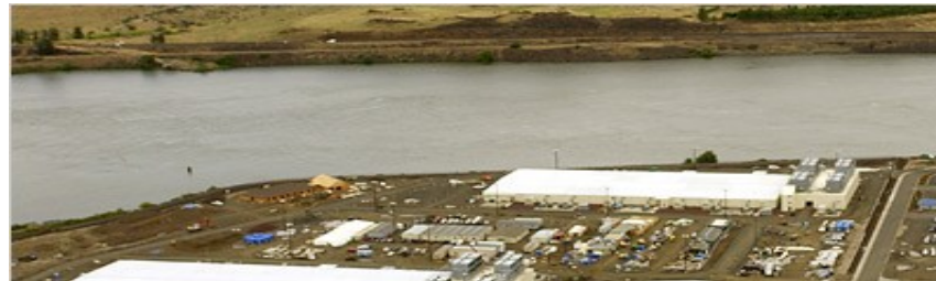
Google data centers The Dalles, OR, USA
