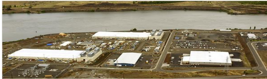
Google data centers The Dalles, OR, USA
