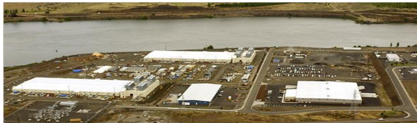
Google data centers The Dalles, OR, USA
